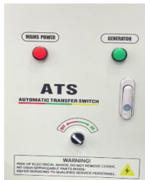
ATS ( Automatic Transfer Switch )
